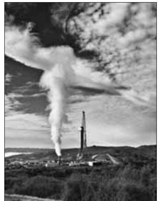
New geothermal well being drilled at the Geysers.
