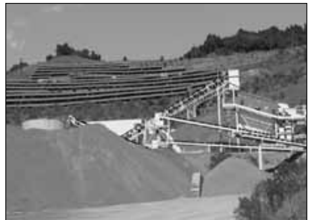
Solar array at BoDean’s Mark West Quarry
